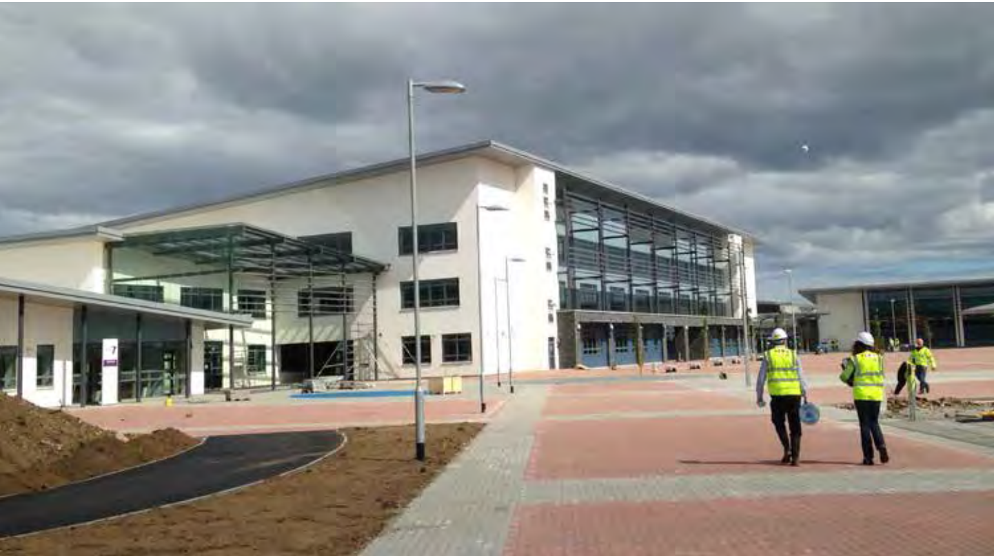
The new school nears completion
